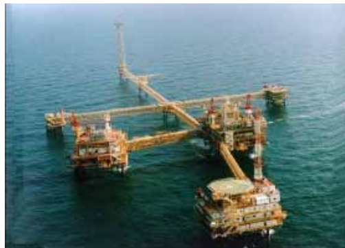
Offshore gas production facility, Qatar
