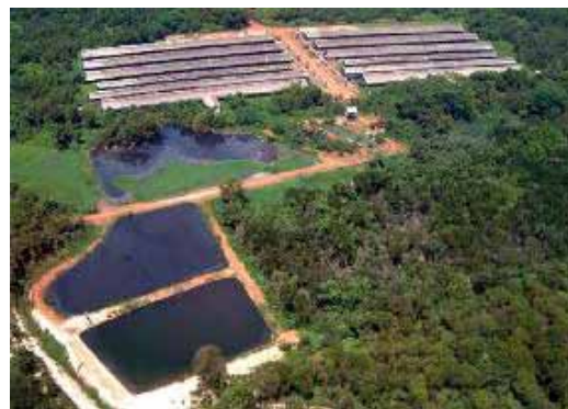
Methane capture and combustion from pig farm, Indonesia
