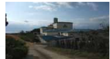
Tokunoshima Clean Center
