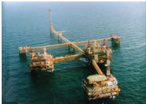
Offshore gas production facility, Qatar
